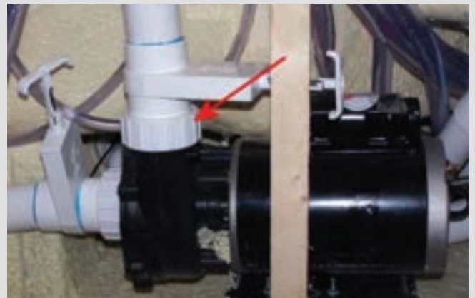
FIGURE 1.9b : PUMP UNION; LOOSEN UP TO BLEED AIR
